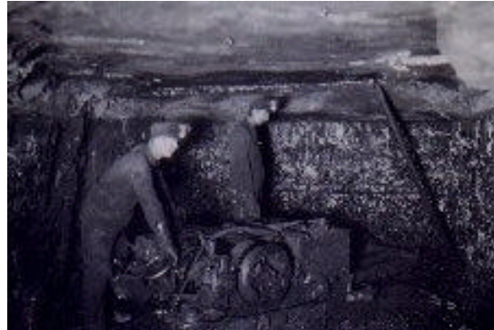
Two miners getting ready to undercut the coal face in preparation for blasting the coal down for hand loading. Cutter probably Jeffrey or Sullivan machine.
