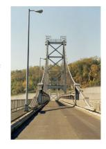
The service life of this Bridge is nearing its end and it is functionally obsolete. Costly repairs will be required in order to extend the Bridge's remaining service life. More importantly, the fact that the structure is a suspension bridge eliminates the possibility of widening the roadway. Given the age of the structure, there will be a continuing concern over the integrity of the main cables, cable anchorages and main piers.
