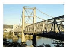
to span the main river channel. The cross-section includes a two-lane roadway and a pedestrian walkway. The west end of the bridge extends into downtown Steubenville, and serves the business district. It is posted with a 5 ton weight limit.
