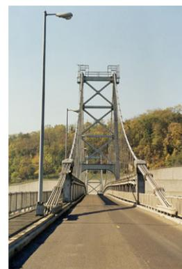
The service life of this Bridge is nearing its end and it is functionally obsolete. Costly repairs will be required in order to extend the Bridge's remaining service life. More importantly, the fact that the structure is a suspension bridge eliminates the possibility of widening the roadway. Given the age of the structure, there will be a continuing concern over the integrity of the main cables, cable anchorages and main piers.
