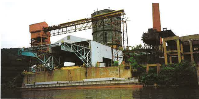
ArchelorMittal Steel Port Facility @ Weirton
