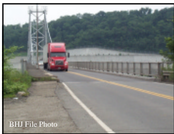
Fort Steuben Bridge
